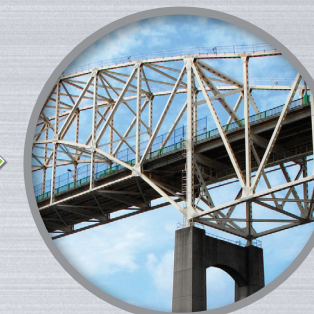
...used in the construction of a new bridge
