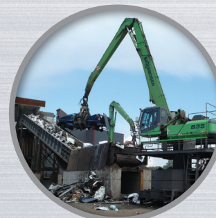
They are inspected, removing any potentially hazardous materials, then shredded
